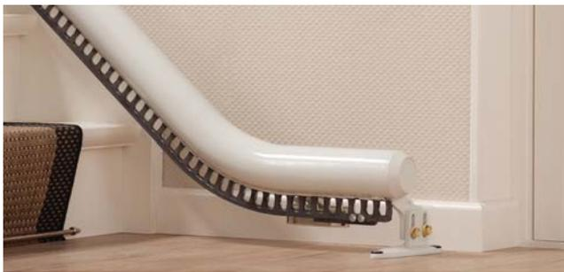
Where you have extra space at the bottom of the stairs the horizontal overrun allows the chair to be parked away from the bottom step.
